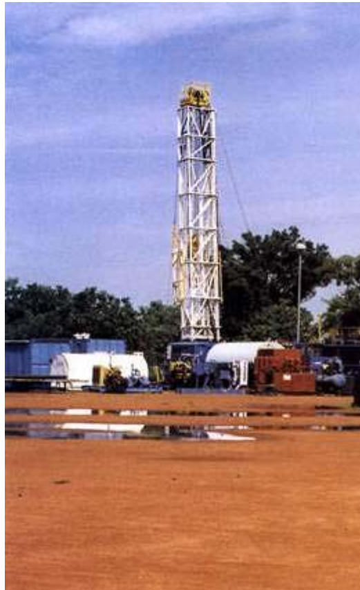
Parker service rig on the Komé field
